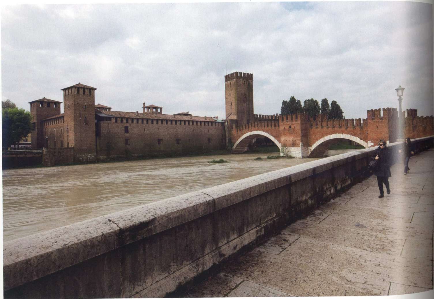
pp. 50-51: General view of the courtyard. The main entrance is on the right and the museum wing is on the left. This page: Exterior view beyond Adige River. Opposite: Walking on the Castelvecchio Bridge toward Castelvecchio Museum. All photos on pp. 50-81 except as noted by Yasuhiro Nakayama / Shinken-chiku-sha.
