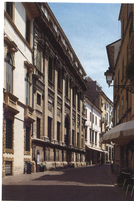
This page left: General view from the street. This page, right: Map drawing by Simone Baldissini. Right page: Original drawing of Palazzo Valmarana (A. Palladio, I Quattro Libri dell'Architettura, Venice 1570, Book II, p. 16). All photo on pp. 142-151 by Noboru Inoue / Shinkenchikusha.
